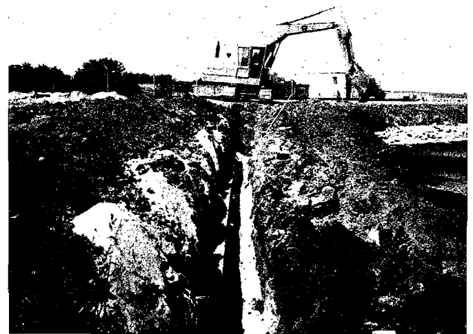
Digging and laying outfall line. Evans, Bierly Hutcheson of Great Bend, Kansas is the engineer on this project.
