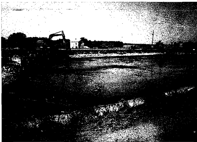
Backhoe installs new outfall line while old lagoon drains.
