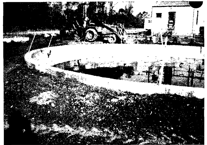
The end is in sight. Structure backfill is complete in spite of tough working conditions. Note that an underground stream has filled clarifier almost to the top with water.
